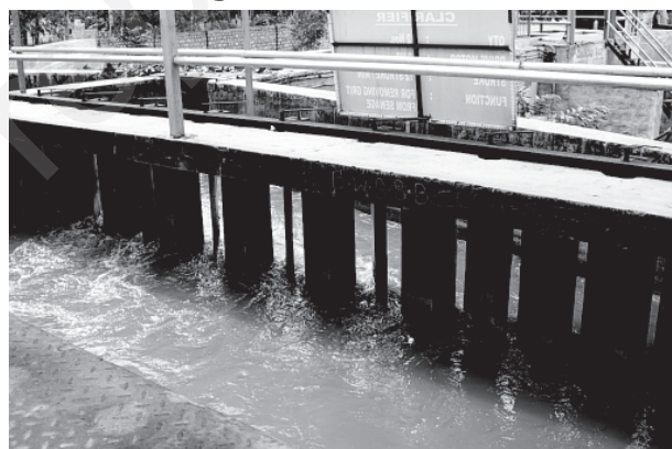
Fig. 18.4 Grit and sand removal tank
