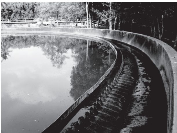
Fig. 18.5 Water clarifier
